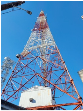
Tower and Antenna
